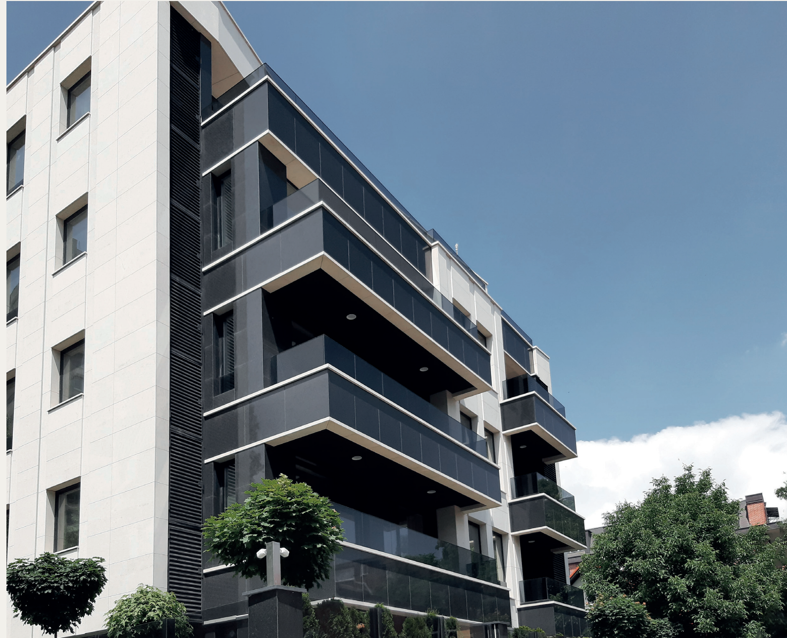
Angola Black, Residential building, Sofia, Bulgaria.
